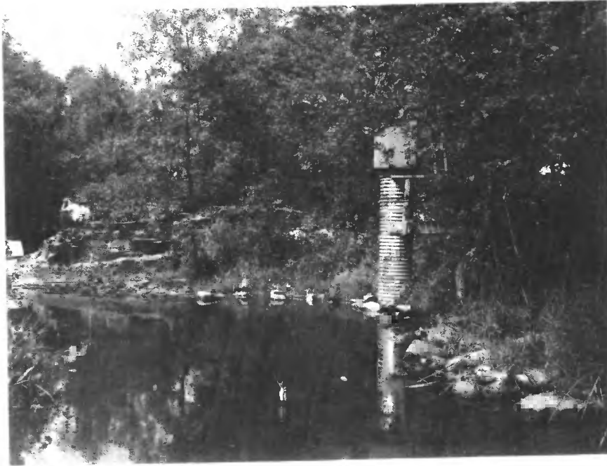
Typical Rockland County Stream-gaging Station
